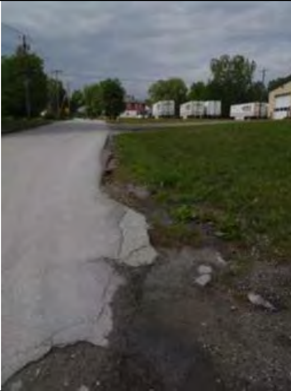
Photo 13. Roadway deterioration and shoulder trenching
