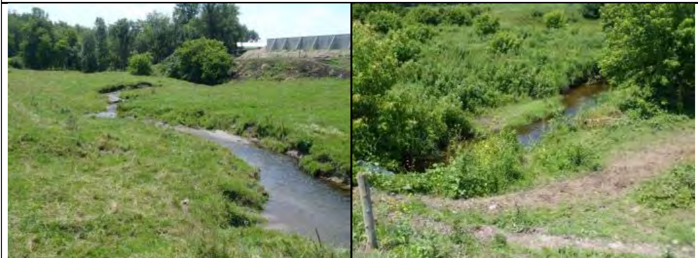
Photo 1. Upstream of culvert
