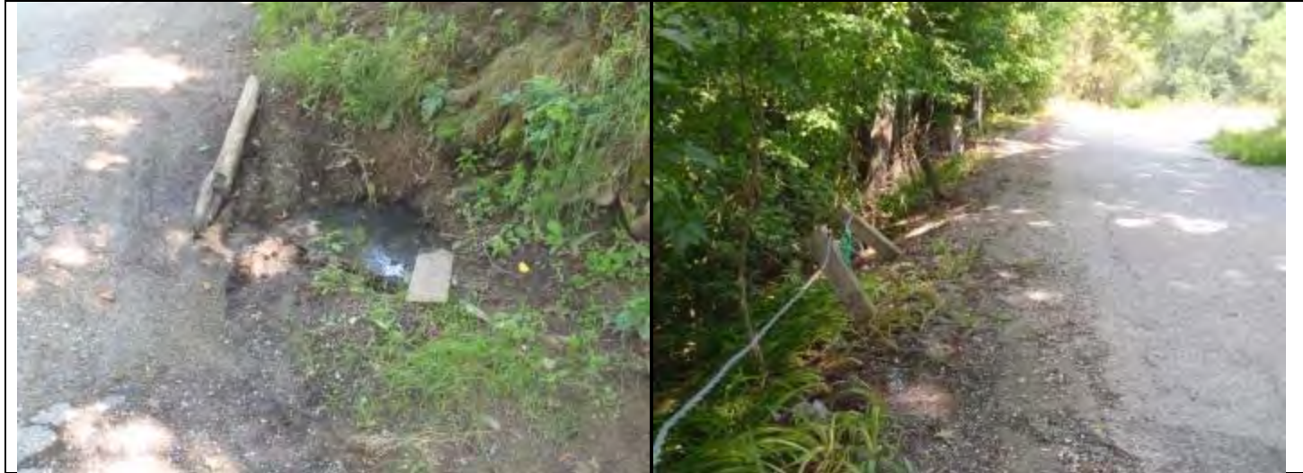
Photo 1. Pool (2' dia.) at culvert inlet Photo 2. Western edge of Church St.
