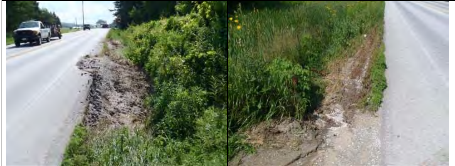
Photo 1. Road shoulder erosion Photo 2. Sediment in ditch
