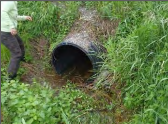
Photo 1. Undersized culvert
