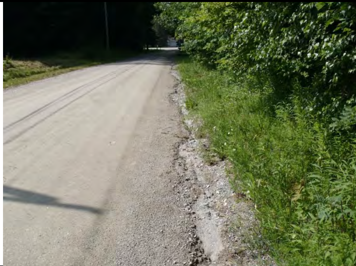
Photo 1. Road-edge erosion
