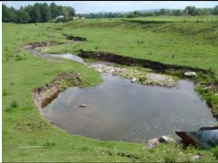
Photo 1. View downstream of culvert Photo 2. Bank slump above culvert
