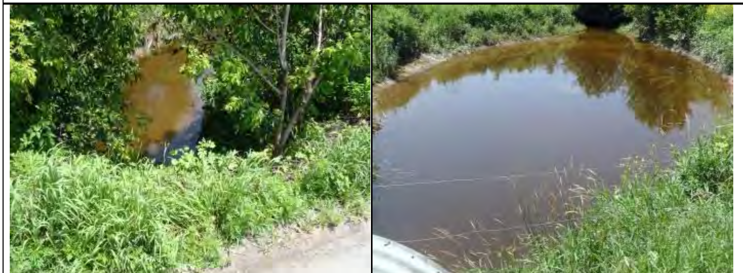
Photo 1. Stream widening upstream of culvert Photo 2. Scour pool downstream of culvert
