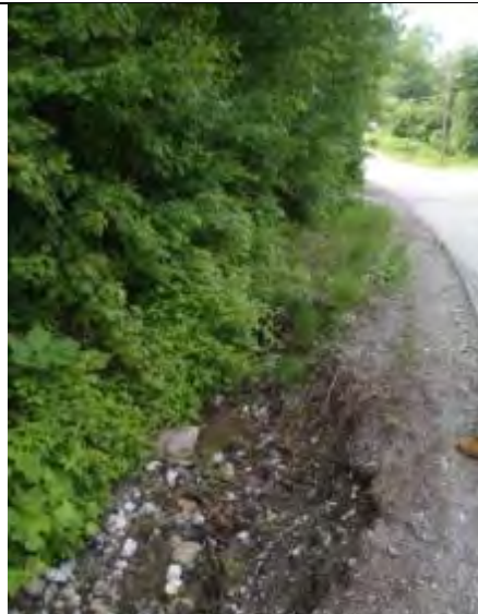
Photo 8 Ditch erosion
