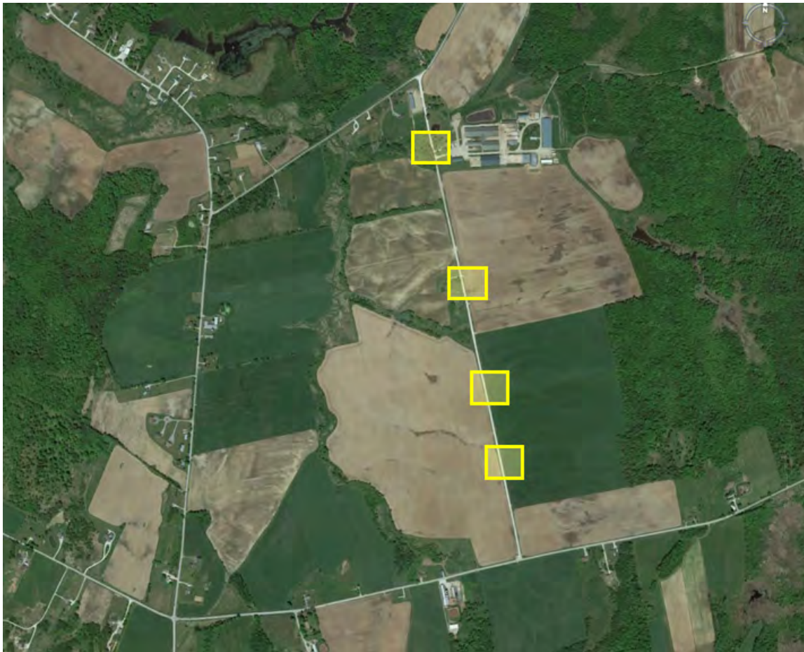
Figure 8. The locations of four undersized culverts along Morey Road.
