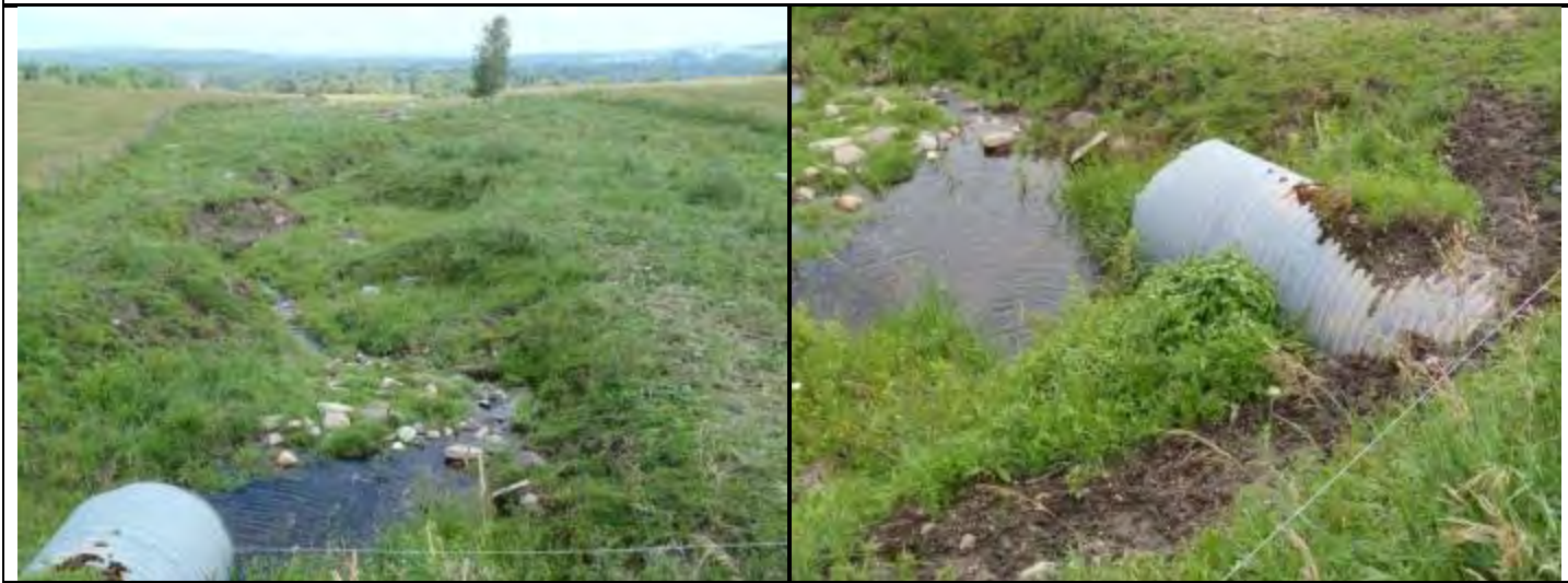
Photo 1. View downstream of culvert
