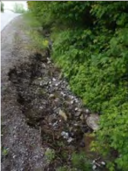
Photo 7. Ditch erosion
