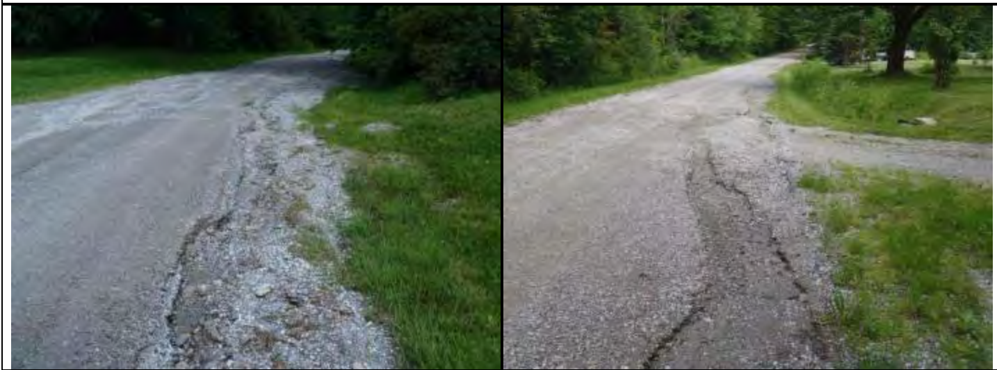
Photo 1. Road-edge erosion
