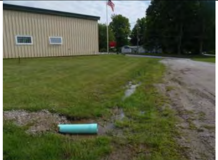
Photo 18. New drainage structure connected to parking lot behind fire station
