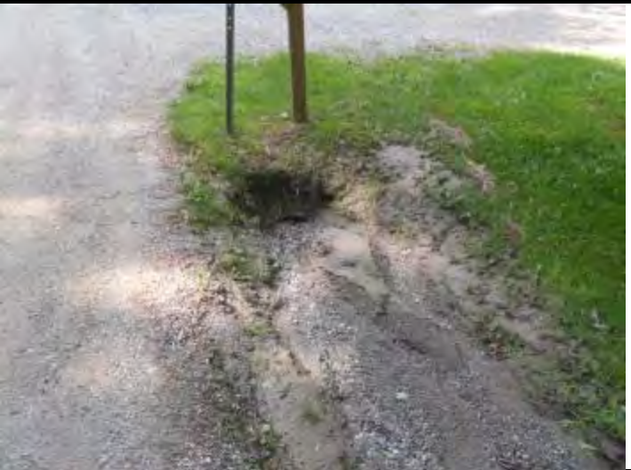
Photo 2. Ditch and culvert full of sediment
