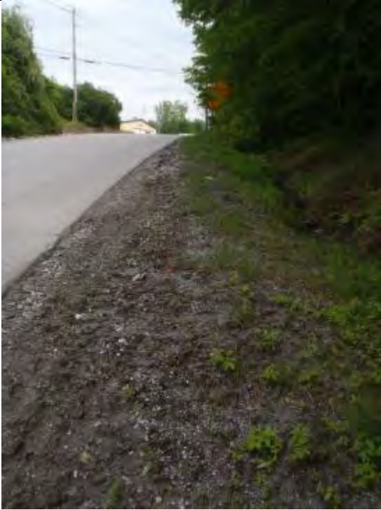
Photo 9 Erosion along road shoulder
