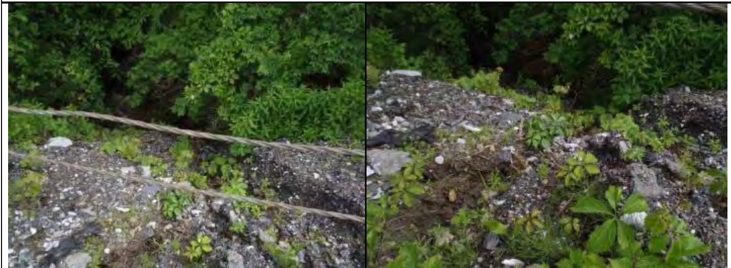
Photo 1. Trenching on road shoulder above culvert inlet
