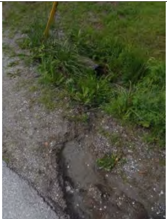
Photo 16. Shoulder trench and overgrown culvert
