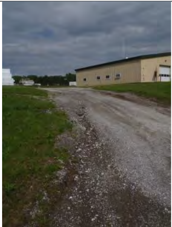
Photo 12. Trenching on gravel driveways subject to heavy truck traffic
