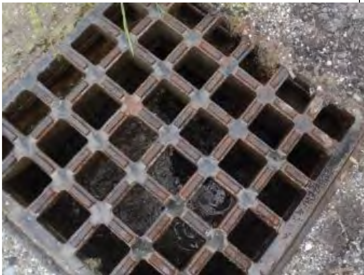
Photo 15. Catch basin filled with sediment
